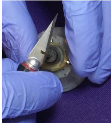
**Figure 4-10 Fixing Exit Tip and Trimming Polyimide tubing**
